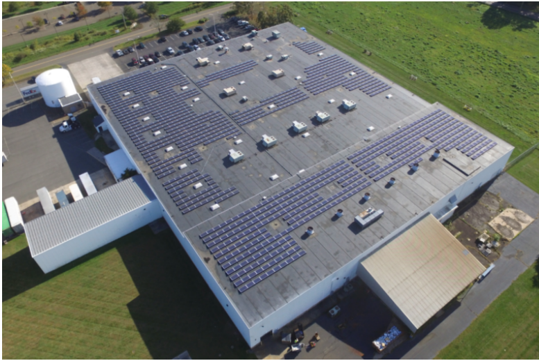
Photos: Vncor Communications, courtesy of Quality Roofing Services
