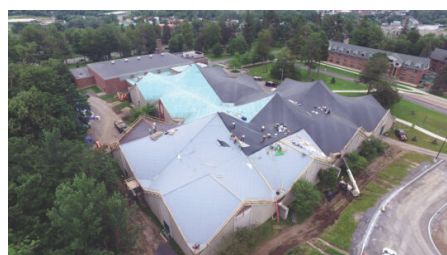
Clarkson University Fitness Center installation of EPDM roof Credit: Carlisle SynTec
