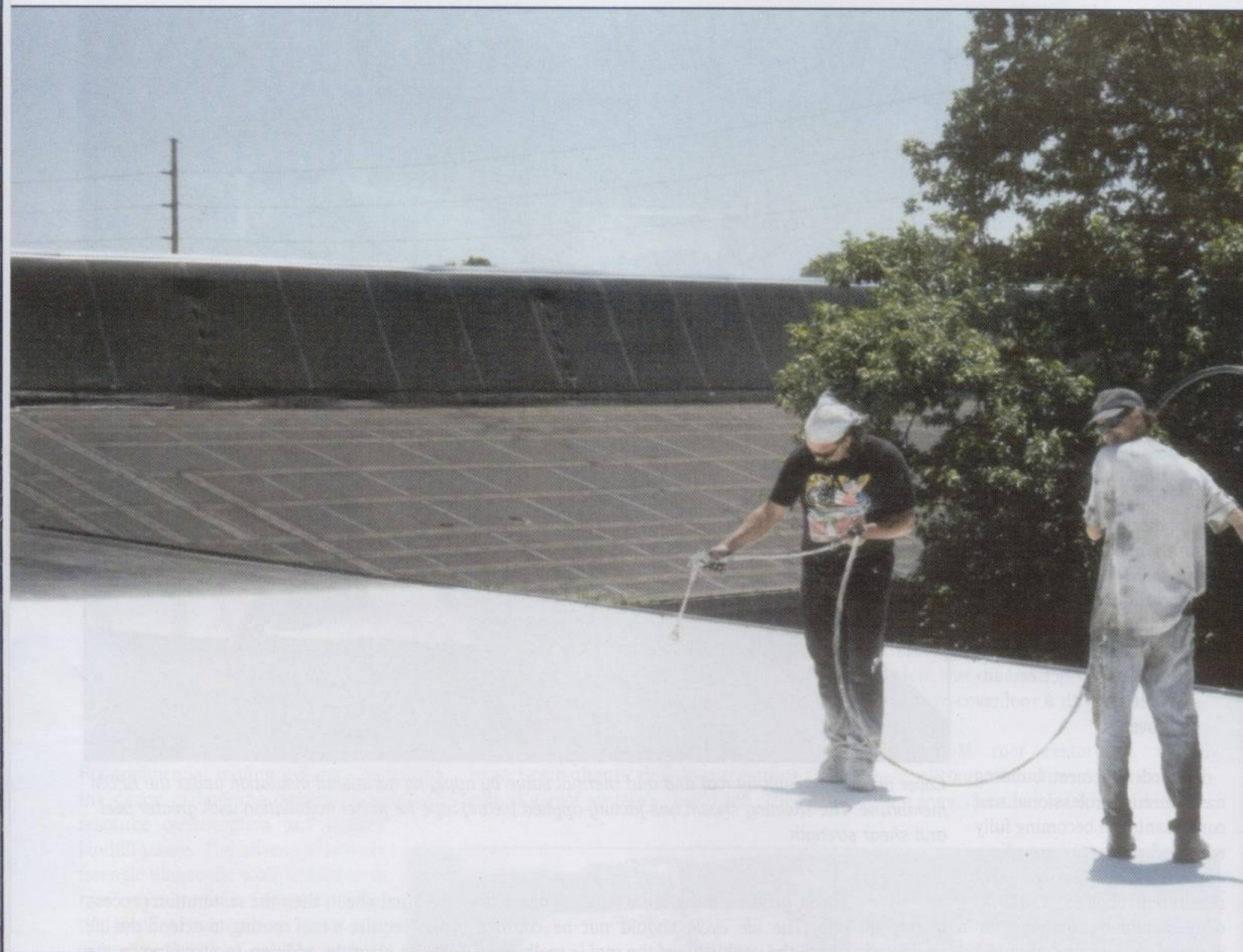
Acrylic coatings such as the one being sprayed on here can help extend the life of an old EPDM roof system (Photo courtesy of United Coatings)
