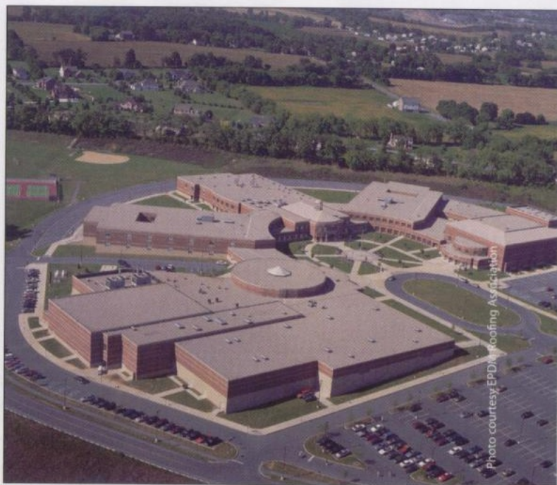
A ballasted EPDM roof tops Parkland High School in Allentown, Pennsylvania. This type of roofing system can offer warranties as long as 30 years and earn up to 12 LEED points. Its cost may also be less than other systems, allowing the difference to go towards upgrades in energy-efficient lighting or windows.
